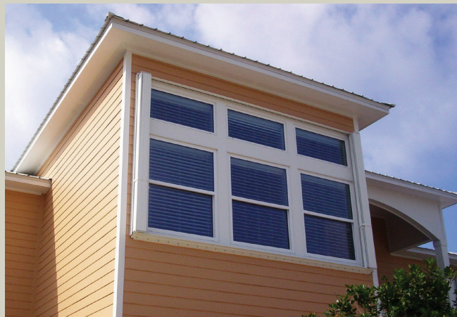
Figure 4-12. Accordion shutter (shown in the open position) installed over large window grouping of a coastal home. The shutter has been installed to allow deployment from inside the home. Source: Roll-a-way/QMI.
