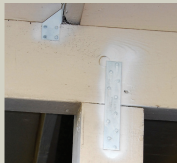
Figure 4-26. In this retrofit example, a hurricane clip attaches the roof structure to a horizontal ridge beam, which is in turn attached to the vertical post with a metal strap. This is an attempt to tie the load from the roof to the foundation, or create the complete load path connection. Note that these clips and straps are in the process of being painted. Source: Hurricane Protection Services.
