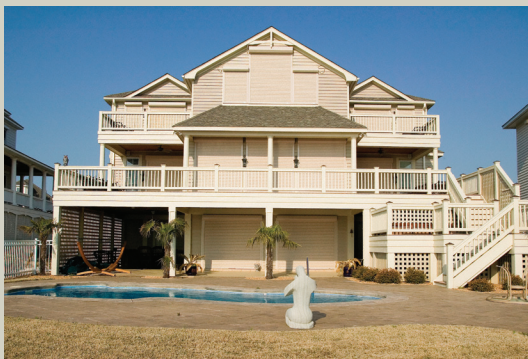
Figure 4-10. Coastal home protected with roll-down shutters on all windows and doors. The shutter is held in place by vertical guide tracks and can be deployed manually or with an integrated electric motor. Source: Roll-a-way/QMI.
