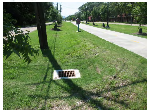
Figure 43. In 2018, the Parish completed the transformation of Canal St. in Metairie by replacing the open drainage canal with underground culverts and installing a landscaped bike and pedestrian path and integrated storm water management. Top is before; middle is a section showing proposed improvements; bottom is after construction of improvements.
