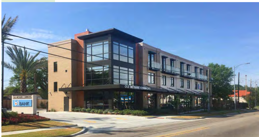
Figure 22. Promoting mixed-use in a more traditional, walkable streetscape is one intent of the Commercial Parkway Pedestrian overlay zoning district, created in 2015. In 2018, Metairie Commons on Metairie Rd. was constructed with apartments above retail and office, using the new zoning standards.
