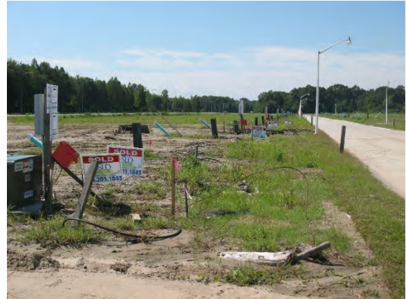
Figure 26. New houses are under construction in the Westwood Crossing Subdivision on the West Bank, where thousands of acres of land are available for development.
