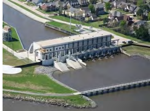
Figure 46. 53 pump stations send storm water into adjacent water bodies through a system of pipes and canals on each bank.
