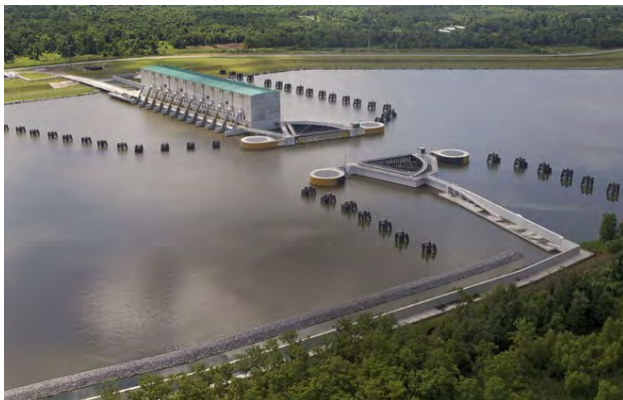
Figure 60. A critical structure in the HSDRRS is the West Closure Complex, the largest drainage pump station in the world and the largest sector gate in North America.
