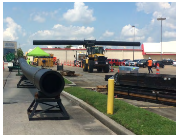
Figure 47. In 2019, an old sewer force main is replaced and upgraded with this new pipe for enhanced performance and safety.
