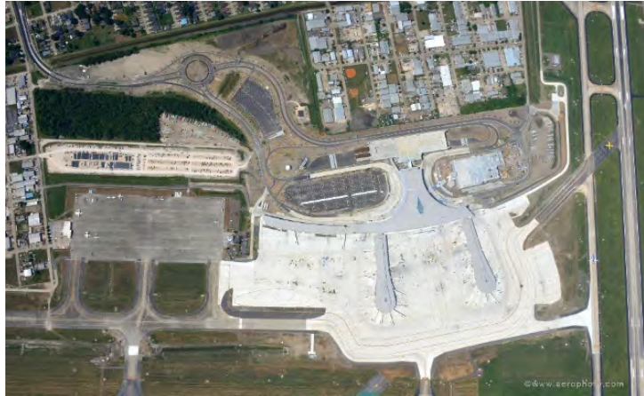
Figure 39. View of the new airport terminal under construction.
